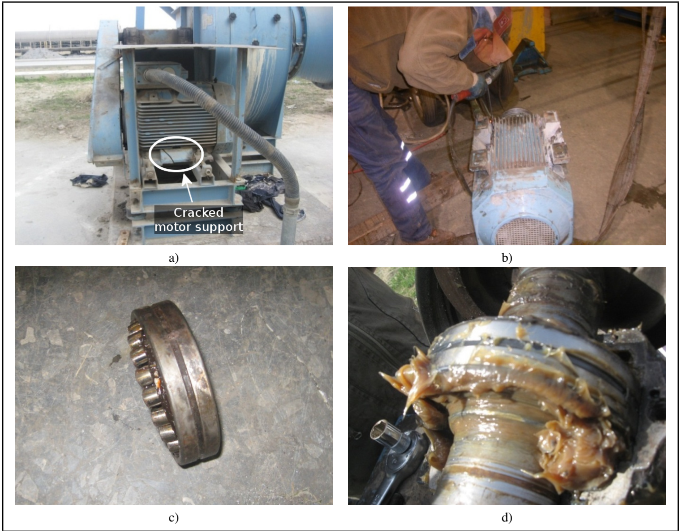
Figure 4. a) Cracked motor support. b) Welding of cracked motor support. c) Damaged bearing. d) Mounting of new bearing.
