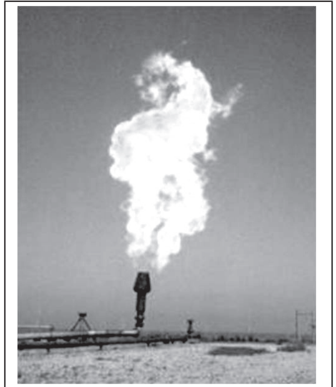
Figure 6. An operating I33 Indair waste-gas flare.
