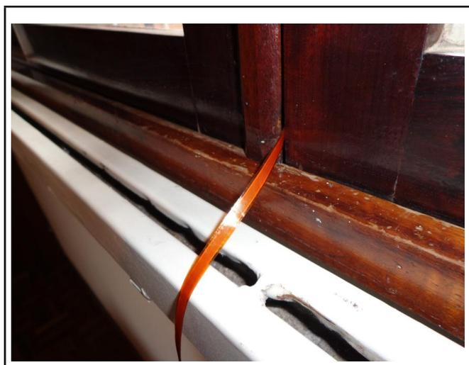
Figure 2. Flat cable through a window.
