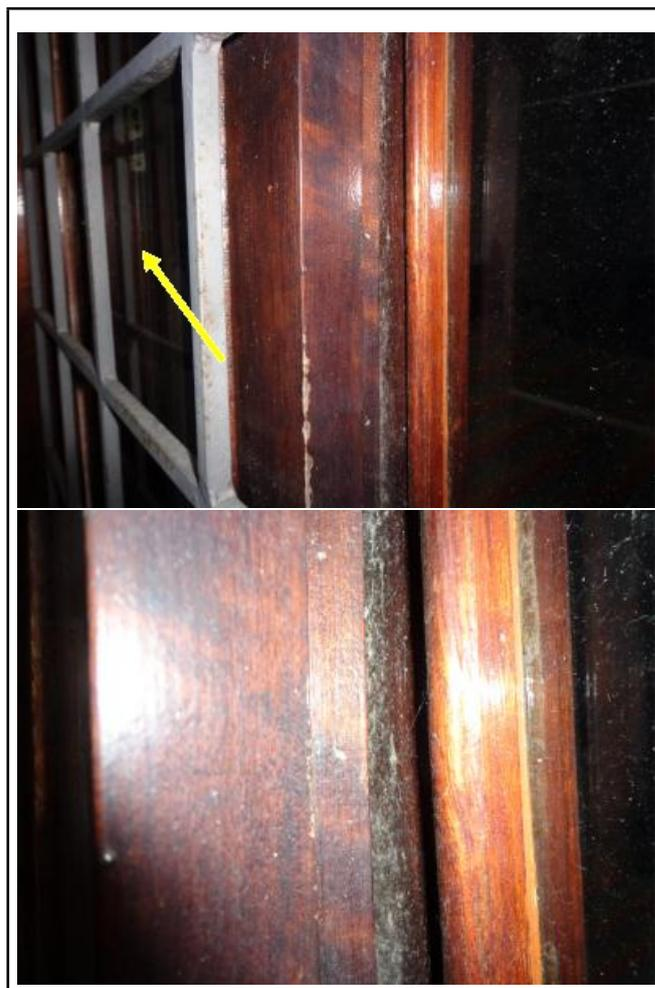
**Figure 5.** Gaps in the window frames of facade 2.
