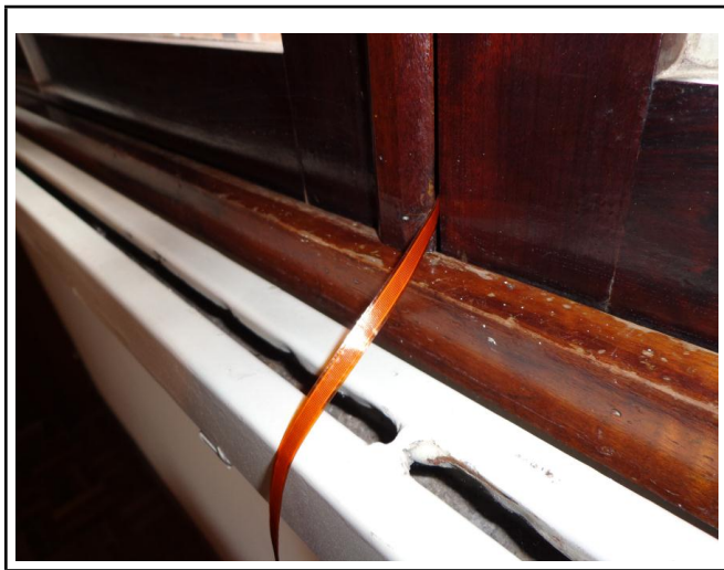
Figure 2. Flat cable through a window.
