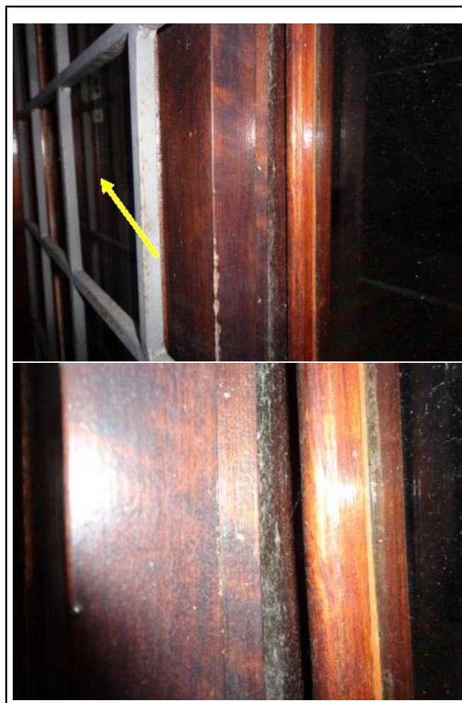
Figure 5. Gaps in the window frames of facade 2.
