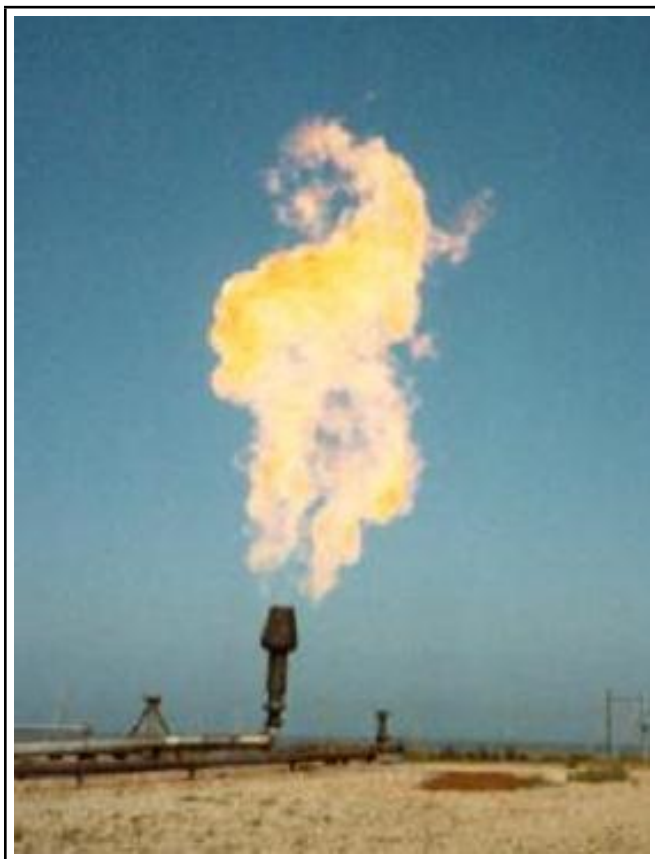
Figure 2. An operating Coanda flare.
